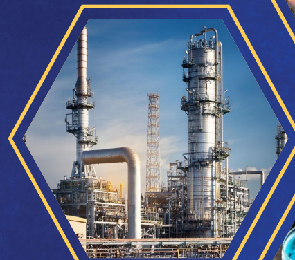
Refineries - Gas & Oil Industries
